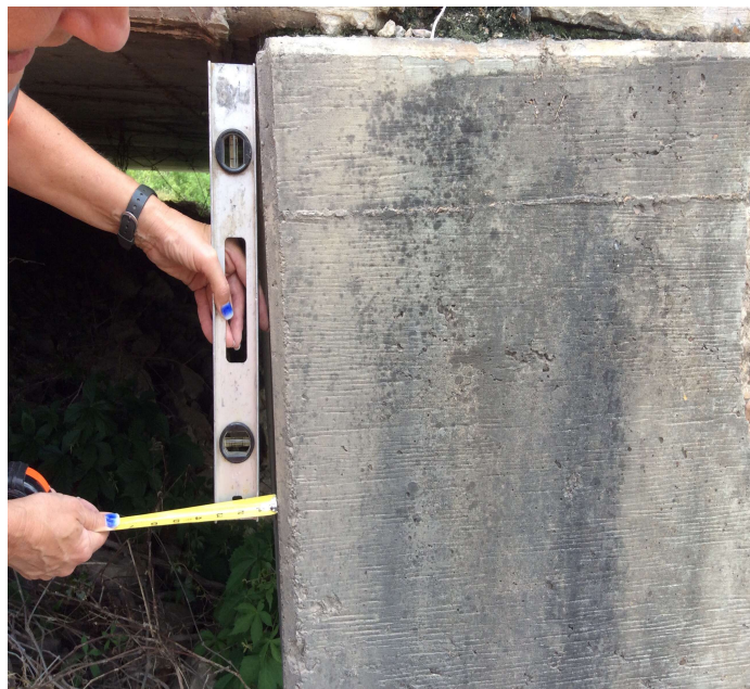
PHOTO 1 Description Bent 1 has rotated back 7/8" in 18".
