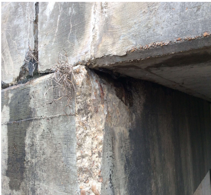
PHOTO 1 Description Bent 1 right end of Cap spall with exposed rebar.
