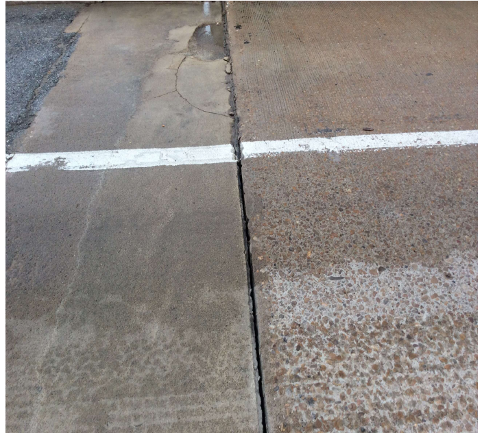
PHOTO 5 Description Abutment 2 right shoulder spalled patch and joint condition.
