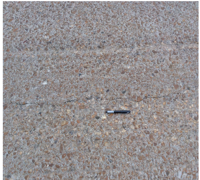
PHOTO 2 Description Span 20 unsealed crack.
