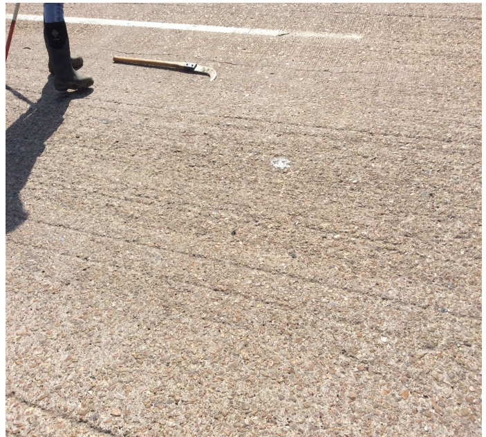
PHOTO 6 Description Typical of Longitudinal cracks to deck @ several spans.
