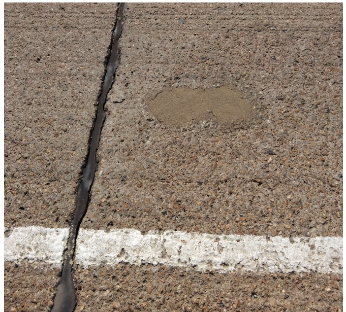
PHOTO 2 Description Spall in right lane at Span 32 with 16" of exposed rebar. Repaired.
