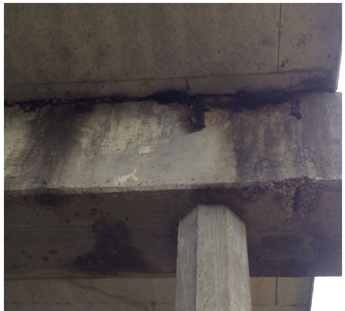
PHOTO 2 Description Bent 2 at Pile 1 spall with 6" of exposed rebar and spall with no exposed rebar at Bridge Seat on ahead side.
