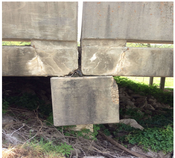
PHOTO 2 Description Bent 1 has rotated back.
