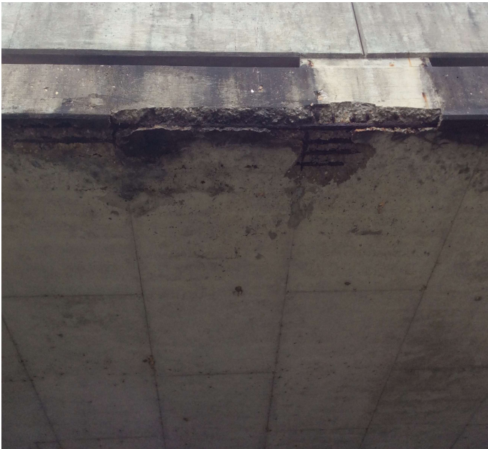
PHOTO 4 Description Right edge of Deck at Span 29.
