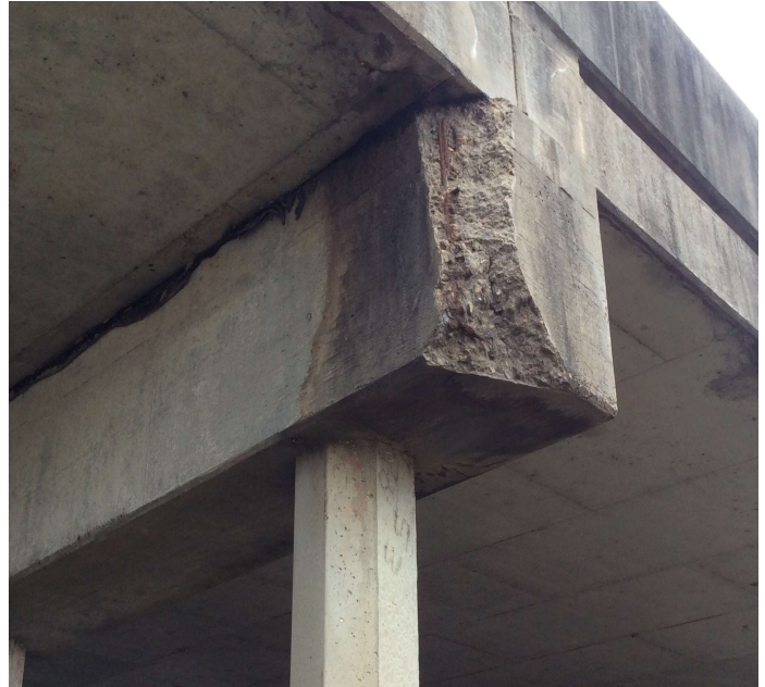
PHOTO 5 Description Right end of Cap at Bent 23.
