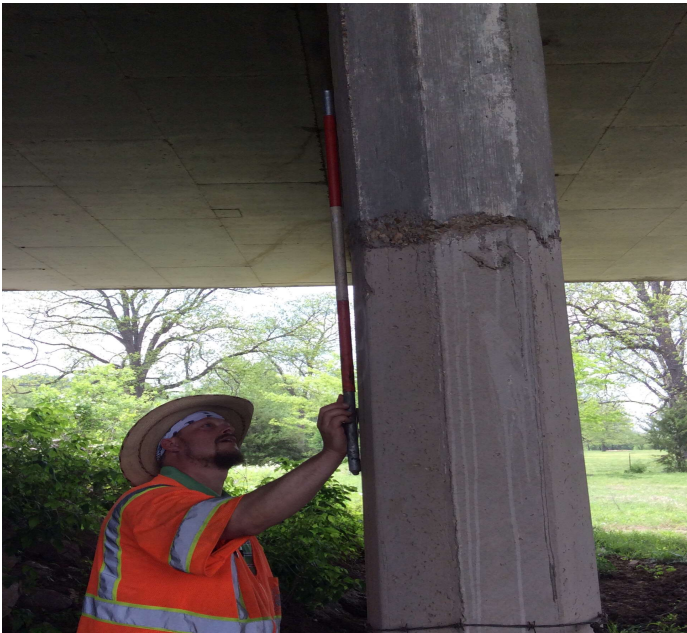
PHOTO 1 Description Bent 1 - Piles 4, 5, & 6 are bowed & leaning back at cracks (cold joints).
