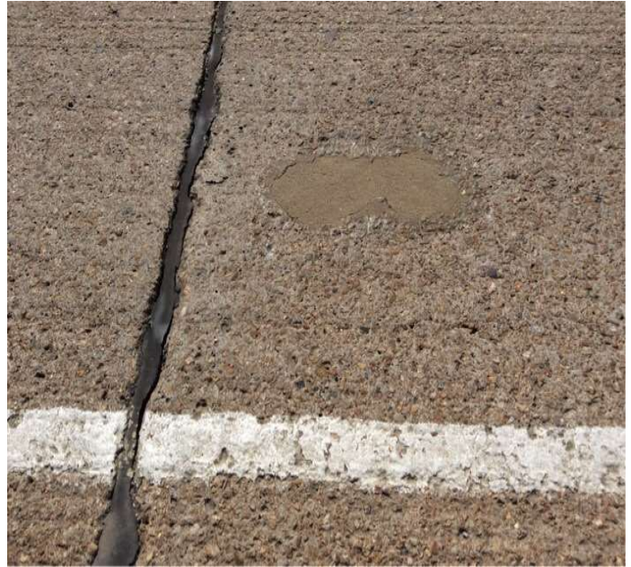
PHOTO 5 Description Spall in right lane at Span 32 with 16" of exposed rebar. Deck spalls Repaired.
